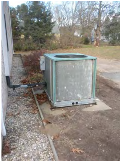
7 ton split system condenser.
