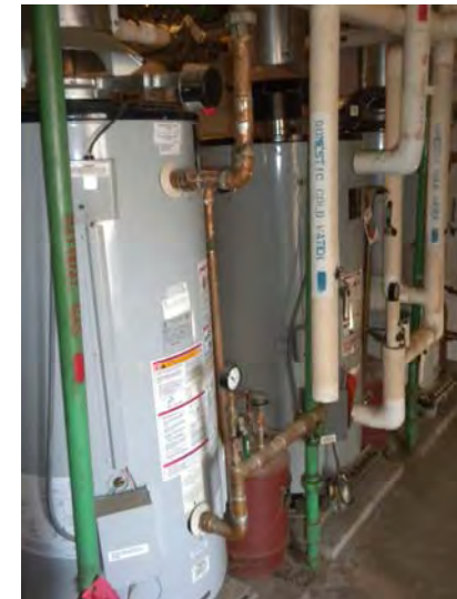
Three natural gas-fired commercial grade domestic hot water tanks.
