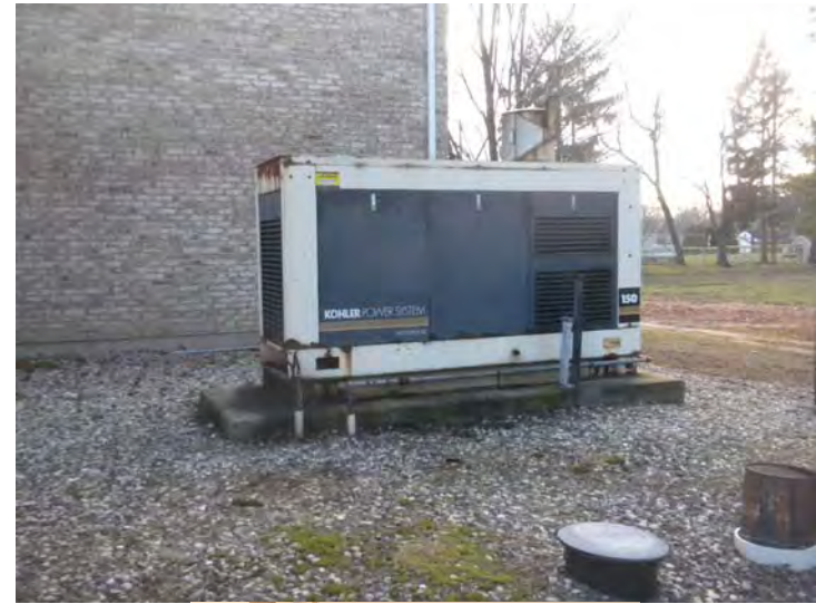
View of the Kohler 150 kW emergency generator.
