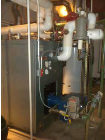
H.B. Smith hot water boiler rated at 1,477 MBH.
