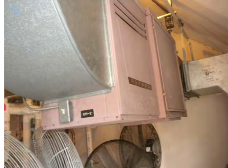
Renzor make-up air unit in the boiler room.
