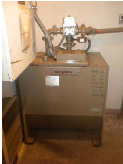
Hydraulic elevator package and controls.
