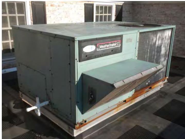
Weathermaker I rooftop unit.
